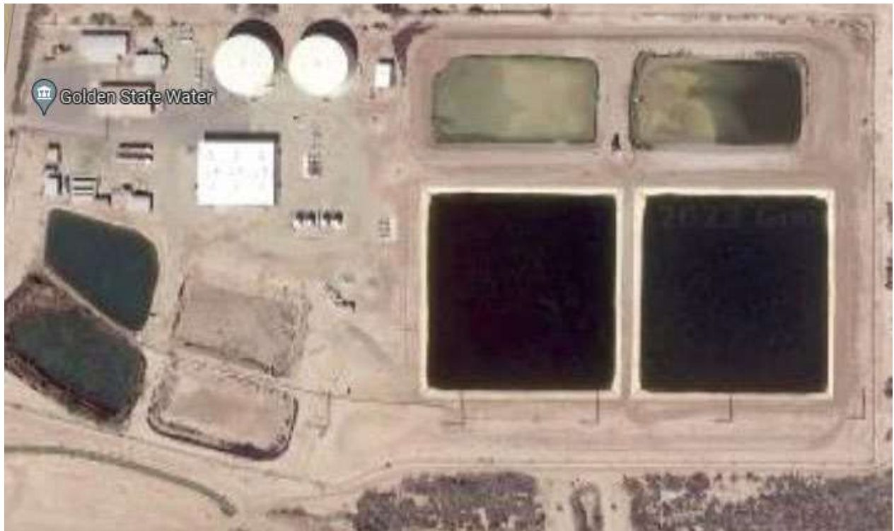
Figure 28: Holabird Plant Satellite Image
